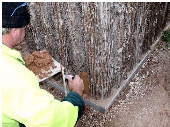
Steven starts the long job of pugging the four walls of Guide Hut
